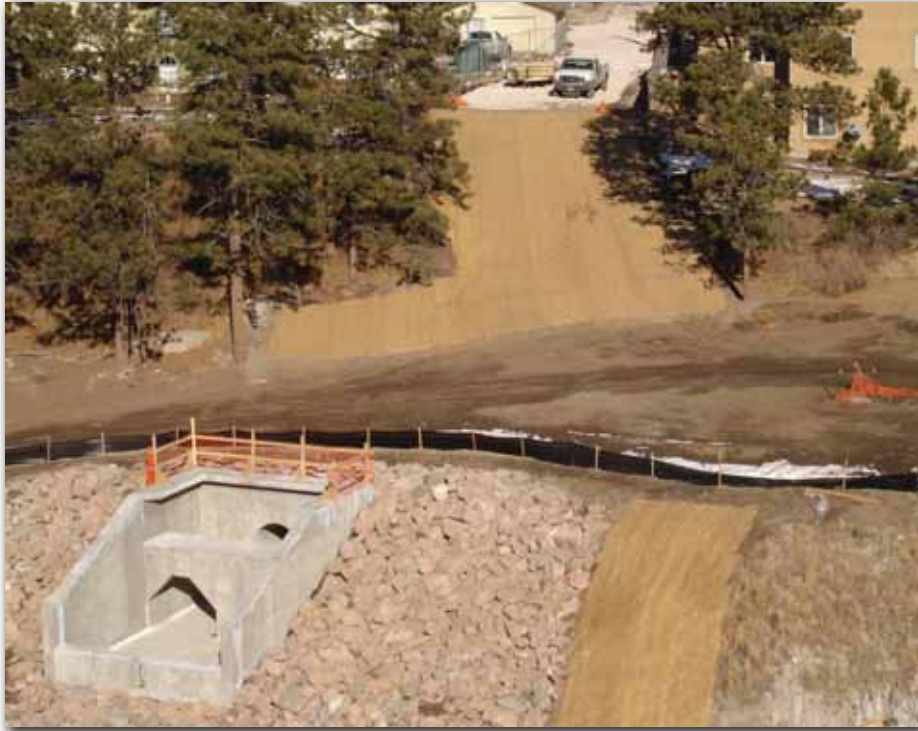
66-inch storm drain outfall structure is now complete.
