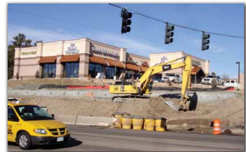
Soil nail retaining wall installation at Relax the Back
